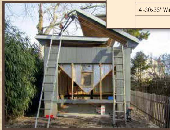
Jacking up Roof
