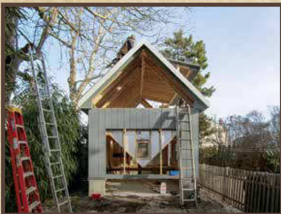
Hinge Roof Under Construction
