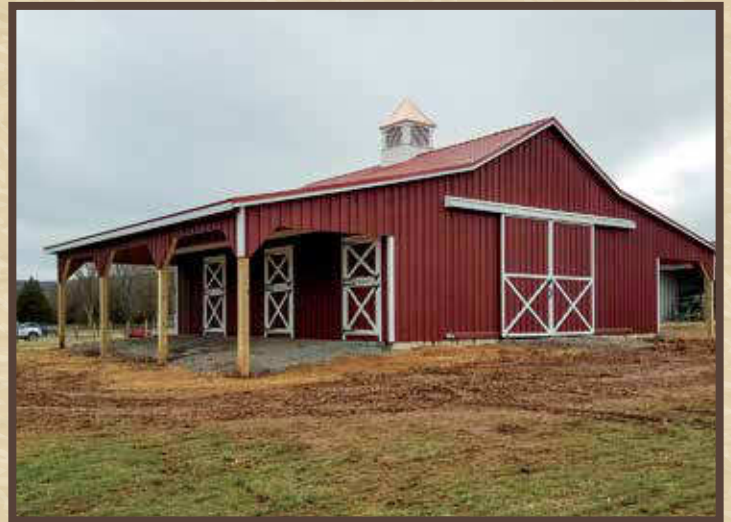
(523) On-Site Build Horse Barn
