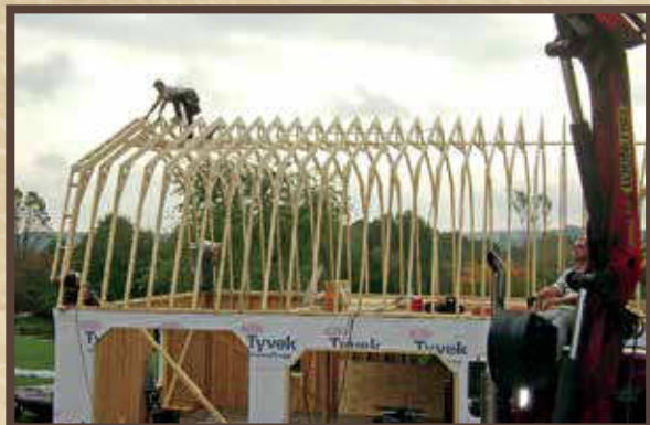
Build On Site
