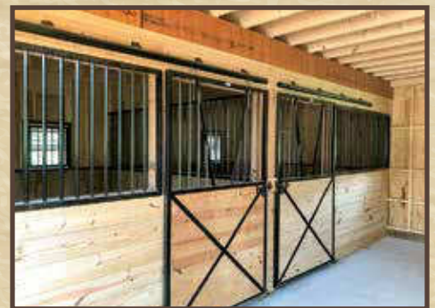
On-Site Build Horse Barn
