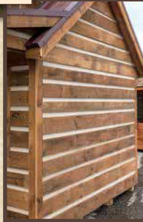
Old Reclaimed Siding with Chinking
