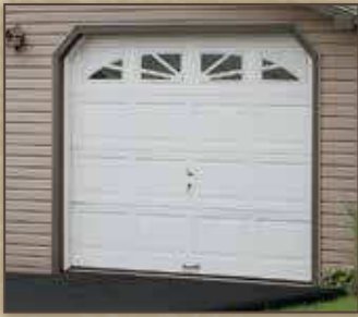
Garage Door with 45 Degree Corners
